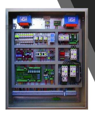
Hydraulic lift controller up to 24kw
